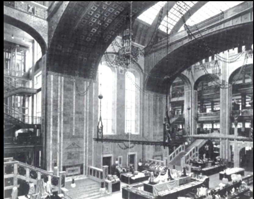
Alfred Messel, Wertheim Department Store, interior
