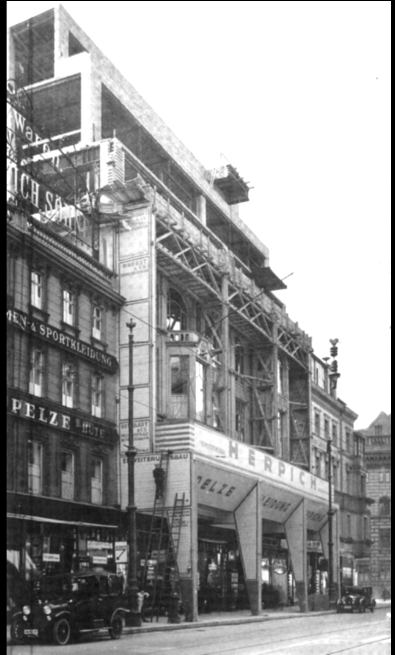
Erich Mendelsohn, C.A. Herpich Sons, Furriers, construction photograph, 1925
